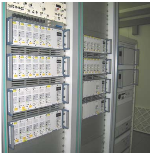
Figure II.6 Group of receivers used in a ground control station for communication on the VHF air radio band. A remote-controlled monitoring system (RCMS) enables the technical service to control and monitor individual receivers (by software via a virtual user interface). For increased operational safety two receivers working simultaneously on two antennas per channel are used for communication between aircraft and air traffic control on the ground. Based on the evaluation of the control voltage (Section III.14) the audio frequency of the RX with the highest received voltage (best signal selection – BSS) is forwarded to the air traffic controllers’ workplace (refer to Fig. II.43). (Company photograph of Austro Control.)
